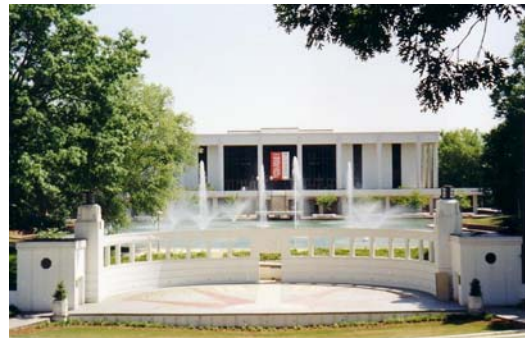
The Madren Conference Center in Clemson, South Carolina.
