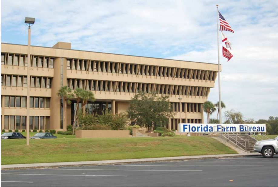
The Florida Farm Bureau building, 5700 SW 34 th Street, Gainesville, Florida.
